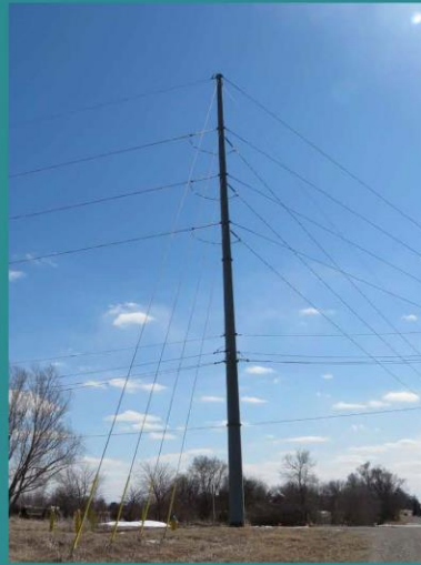
Typical 161kV Fully Guyed Deadend Transmission Pole
